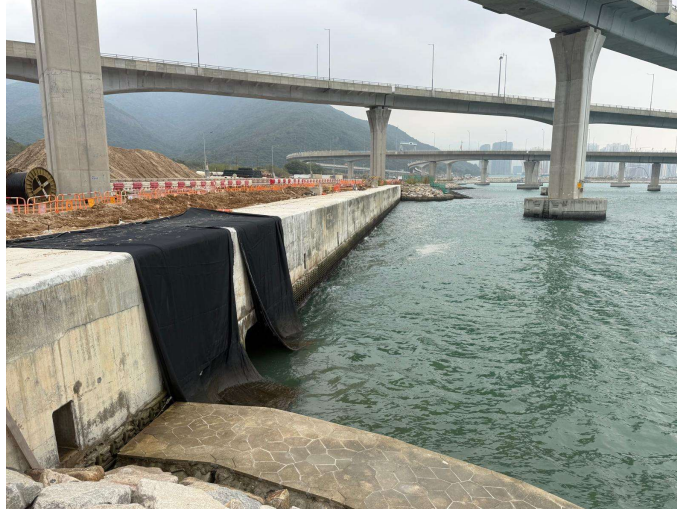
General View of Vertical Eco-shoreline
