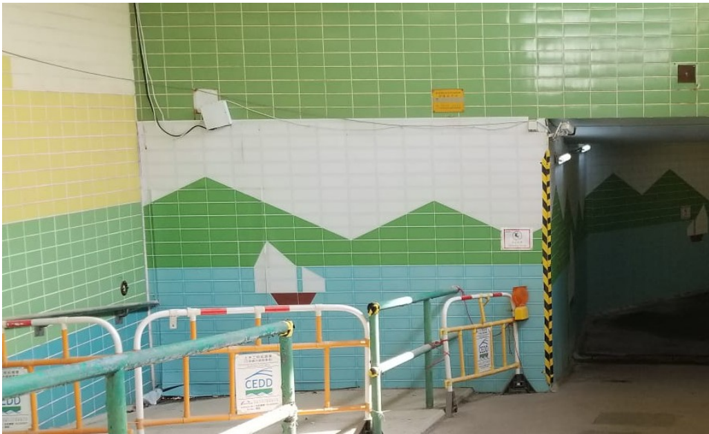
Photo 3 – Erection of site hoardings in unobtrusive colours
